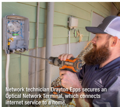
Network technician Drayton Epps connects a new customer.
